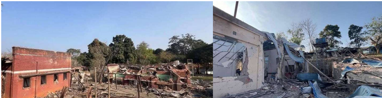
Kyaukme hospital buildings destroyed by SAC bombs
