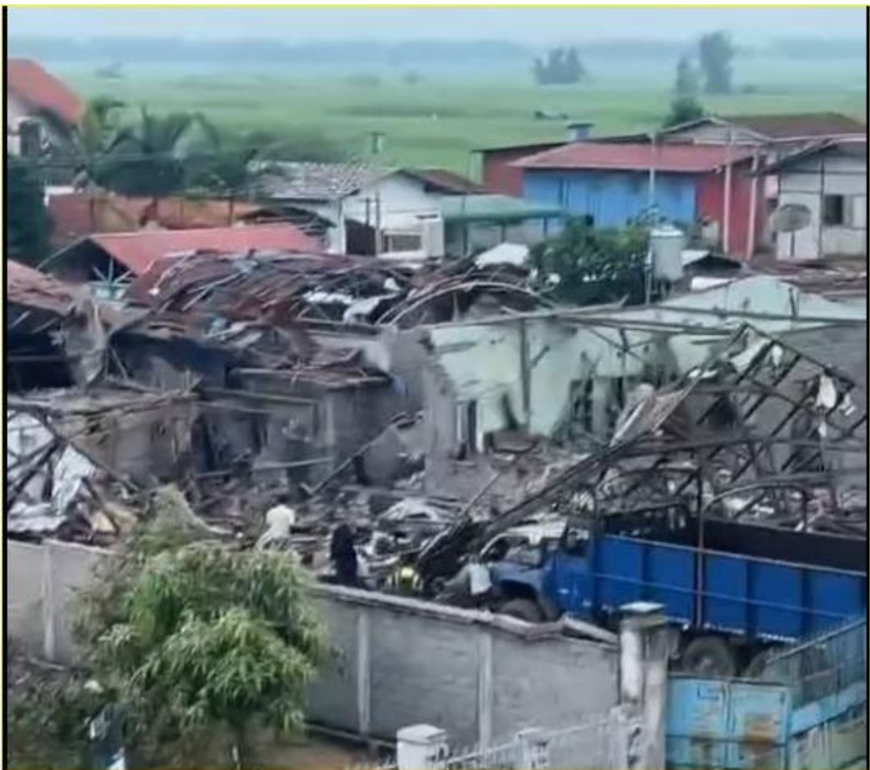
Damage from 500 pound bomb dropped by SAC aircraft in Namkham town
